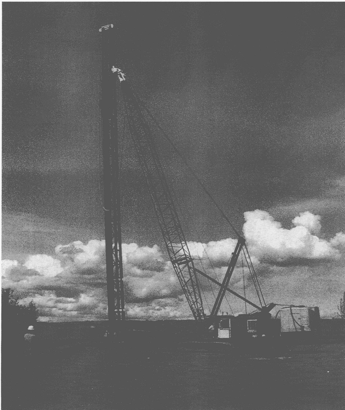
Figure 36-8 The pile driver setup.
