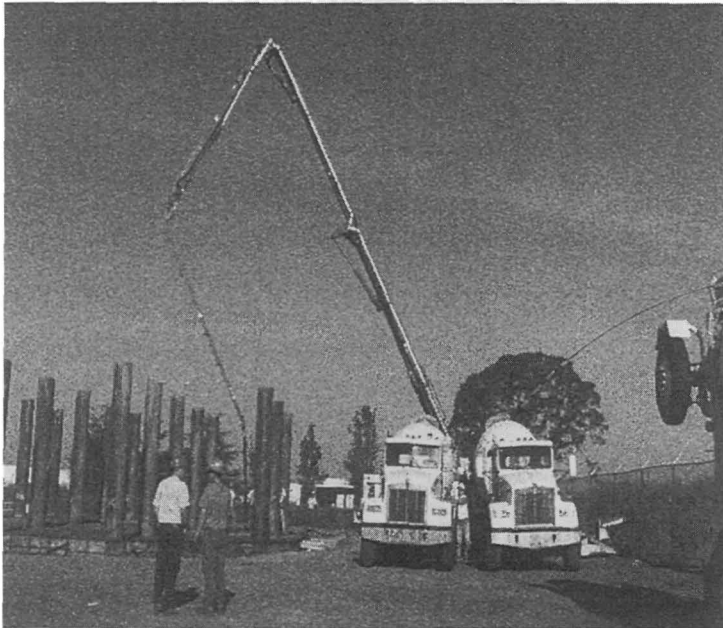
Figure 47-3 Two trucks are shown in position to load the pump hopper.
