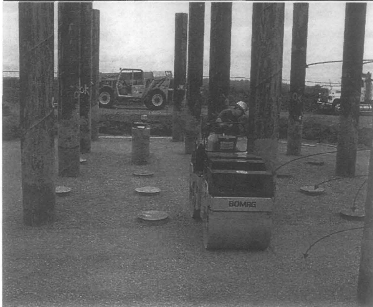
Figure 47-1 Compacting the gravel housekeeping mat.
